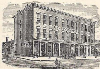
ORIGINAL CENTRAL HOTEL BUILDING
