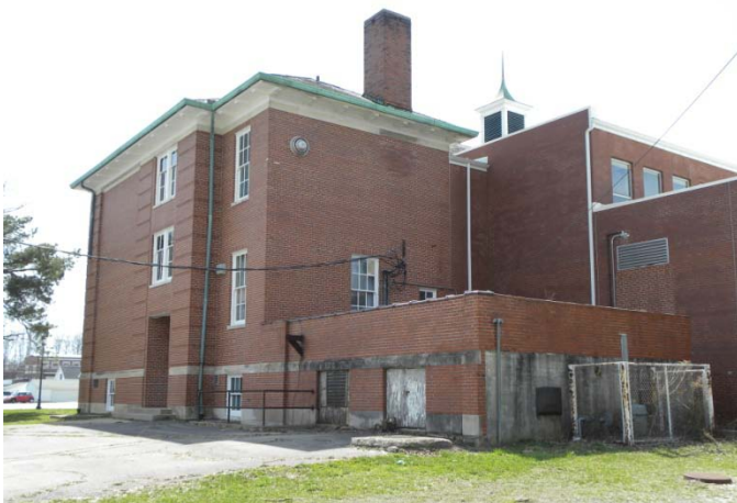
N/E corner boiler room (structure behind is new gym)
