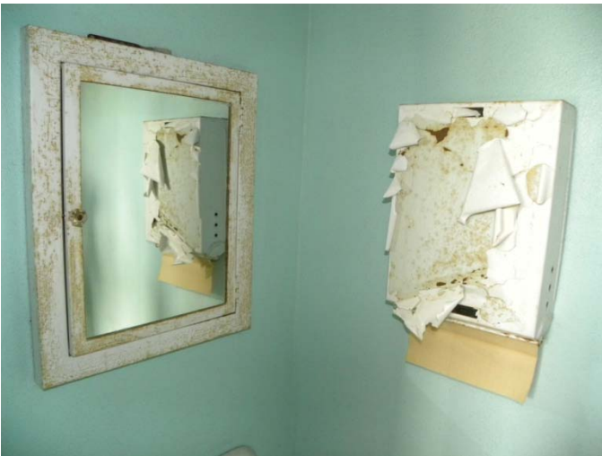
Above the sink
