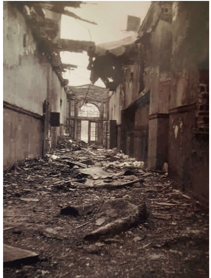
North Hall, Looking West
