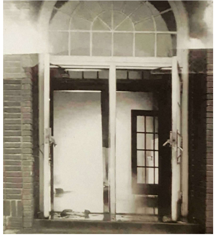
North (Back) Entrance
