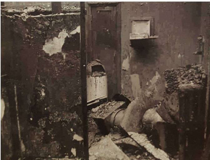
Inside a Restroom
