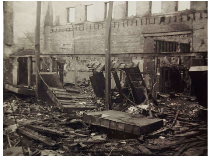
Gymnasium Looking Northeast
