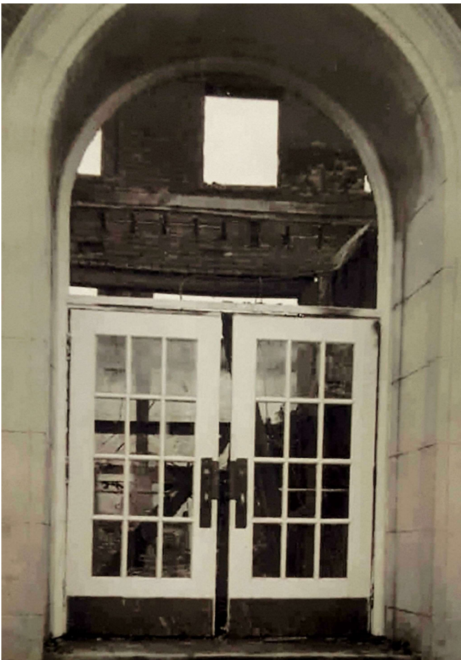
Front Entrance (East Side)
