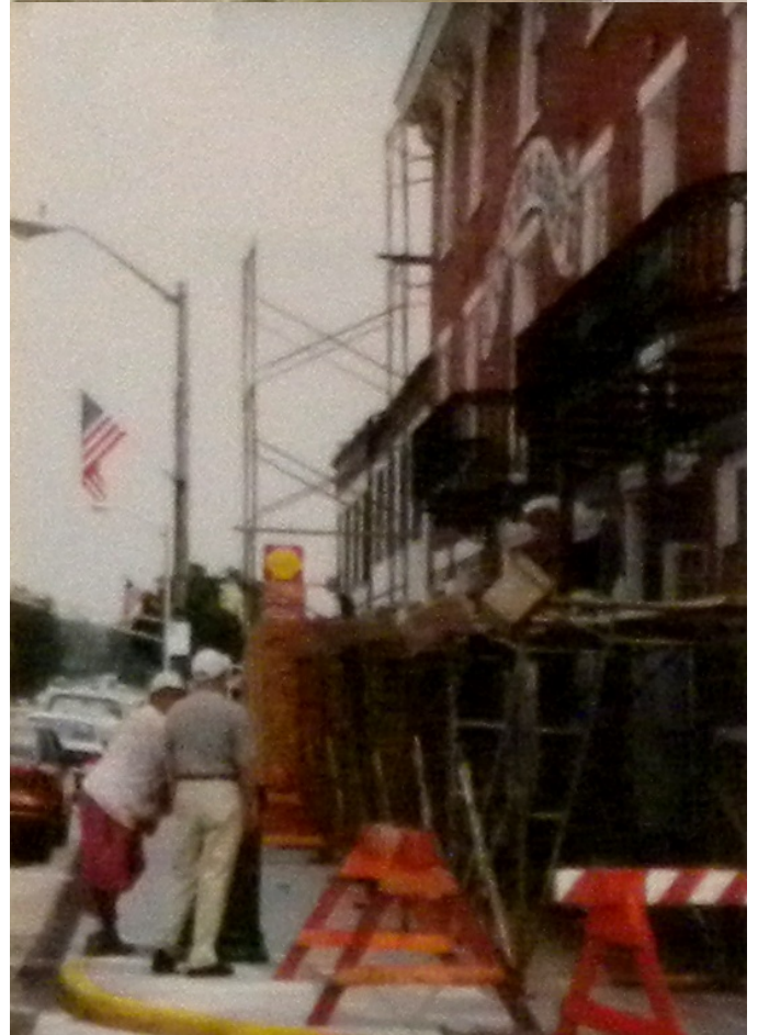
Summer 2001 Masonry Work
