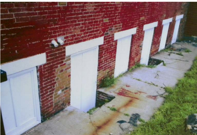
These west side Vinton House doors originally opened directly onto the canal bank allowing goods, warehousing, exchange, and offices to conveniently serve the canal boat clientele
