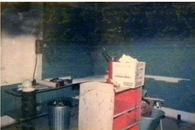
Kitchen, First Floor East Side
