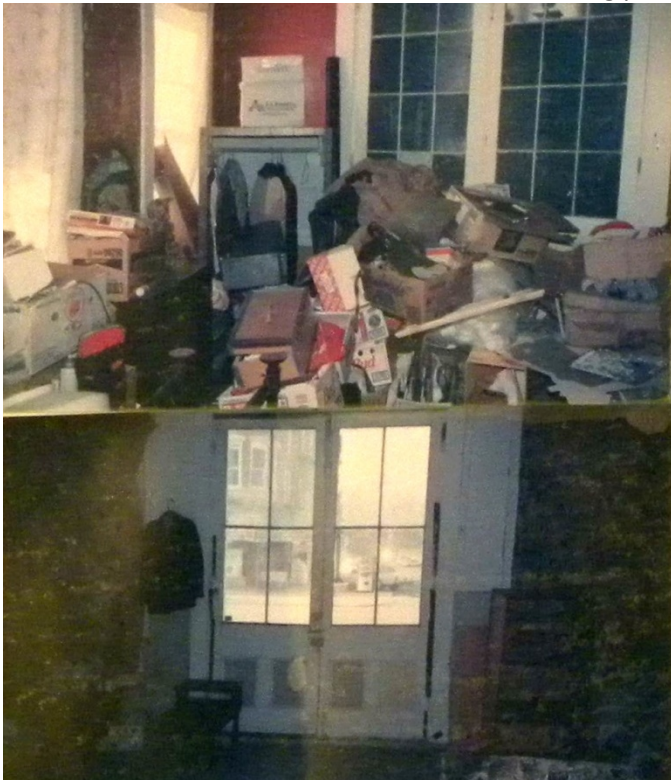
First Floor, West Side
