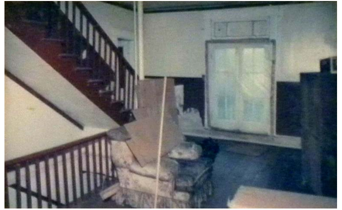
Second Floor Landing
